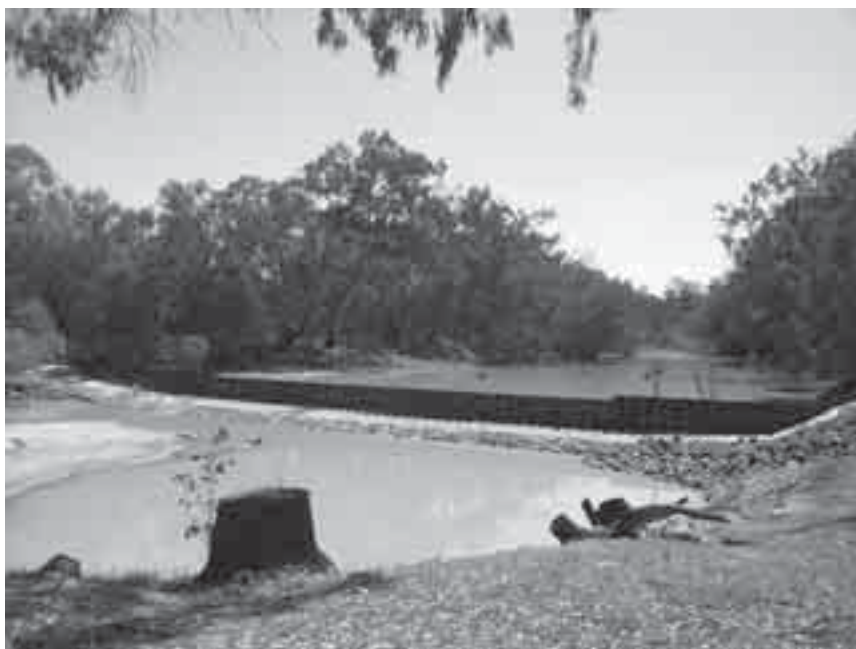
Bifurcation weir on Balonne Minor River at Hastings
