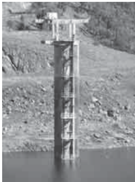
Glenlyon Dam inlet tower
