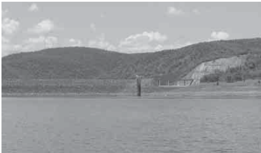
Glenlyon Dam (looking toward embankment, inlet tower and spillway)
